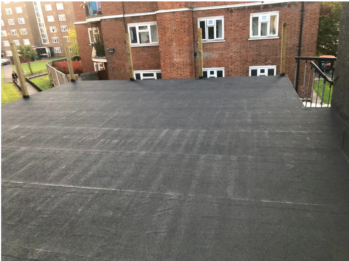
Completed roof, finished with acoustic felt:
